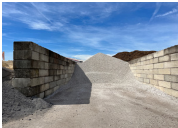
Grondbank, Meppel, the Netherlands
