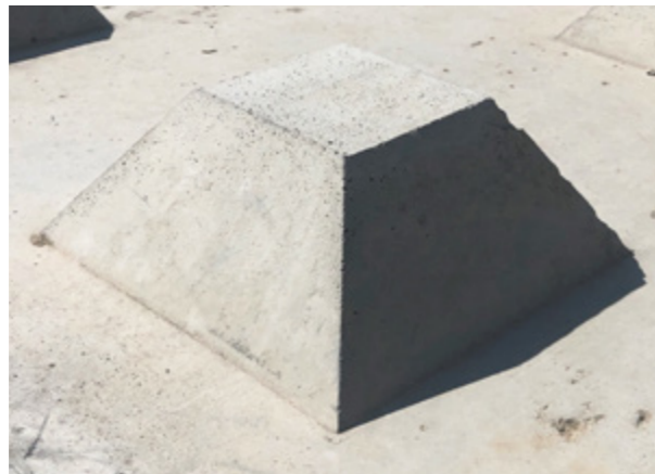
Interlocking element of a concrete block
