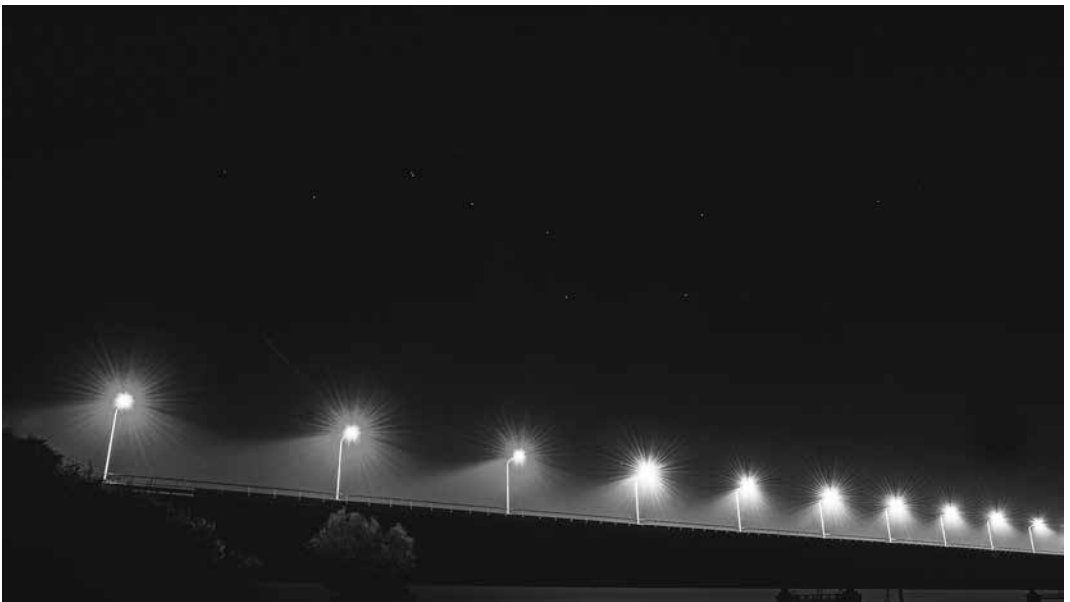
Figure 10 The red streetlights use a spectrum that is friendlier to both bats and moths. © Compass. https://www.compass.nl .
